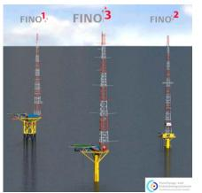
Fig. 1: Mast designs with different foundations. [Source: FuE-Zentrum FH Kiel GmbH].
